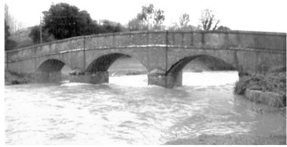
GOSFORD - Gosford Bridge – SY09 NE 3/65 Gosford Bridge was rebuilt after the old bridge was washed away on October 4th 1824. Present bridge is very like the original with 3 segmental arches.
