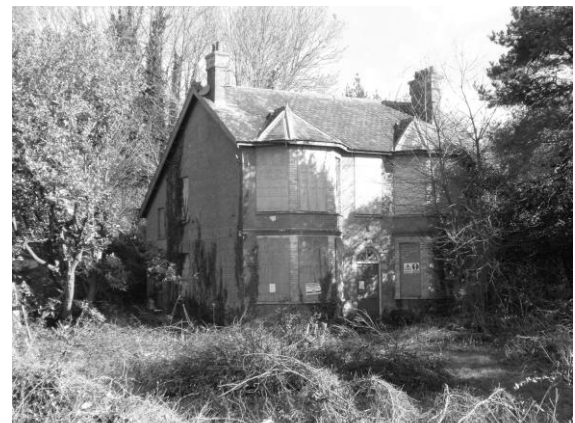
MILL STREET – Factory House (to SE) – SY09 NE 1/24
