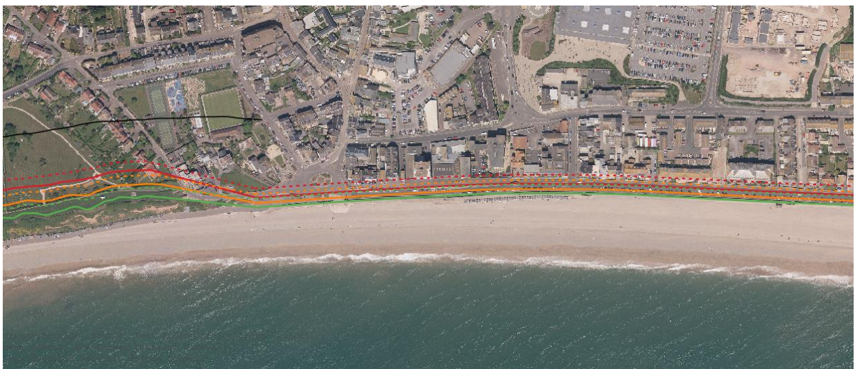
Figure 3-5. Aerial image of Seaton showing the line positions for the short (green), medium (orange) and long term (red). While the lines are identical (in colour scheme) to the cliff sections they are saved as a separate layer because they represent coastlines backed by sea defences (SD). The 100 yr SMP line is also shown where available (black).
