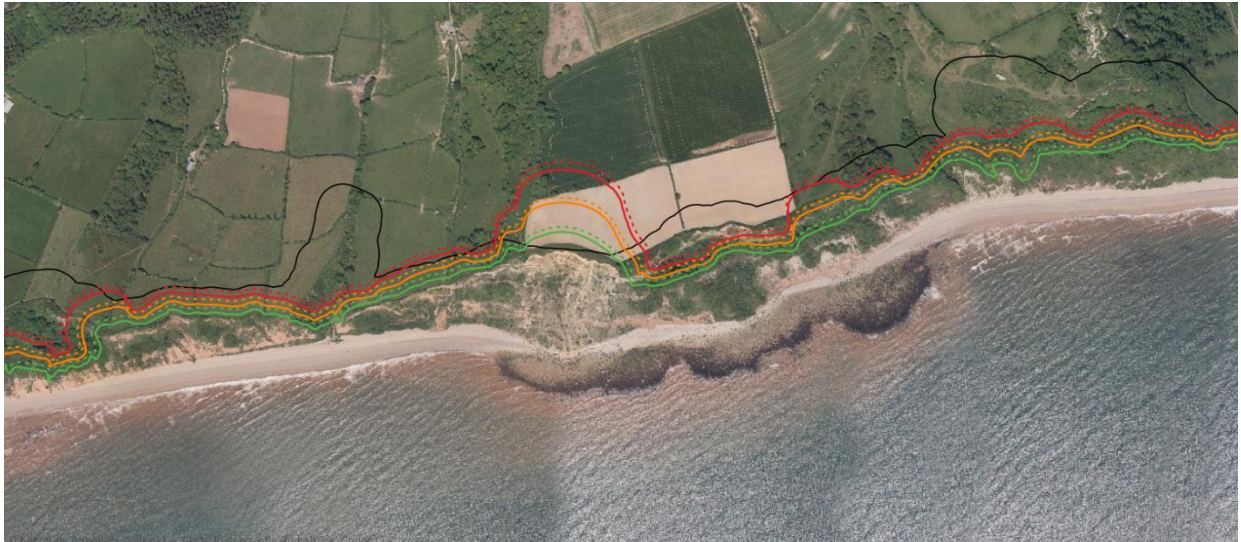
Figure 3-4. Aerial image of a section of East Devon coast with the predicted cliff line positions for the short (green), medium (orange) and long term (red). The dashed lines indicate the ‘buffer’ for each epoch. The 100 yr SMP line is also shown (black).
