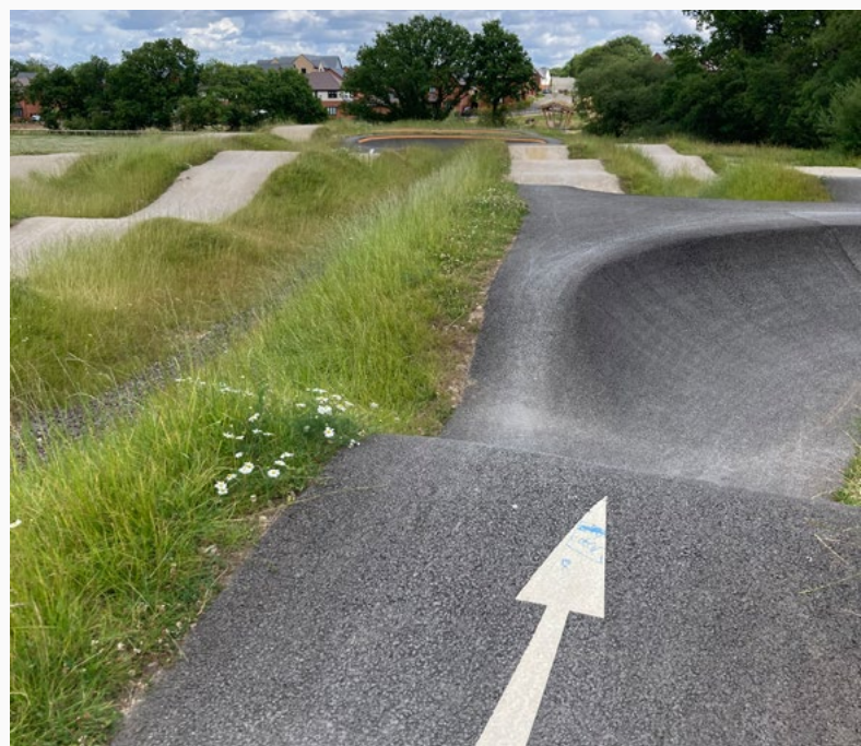
Pump track at Blythe Valley Park, Solihull.
