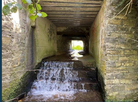
Downstream face, looking upstream:
