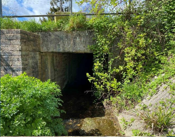
Upstream face, looking downstream:
