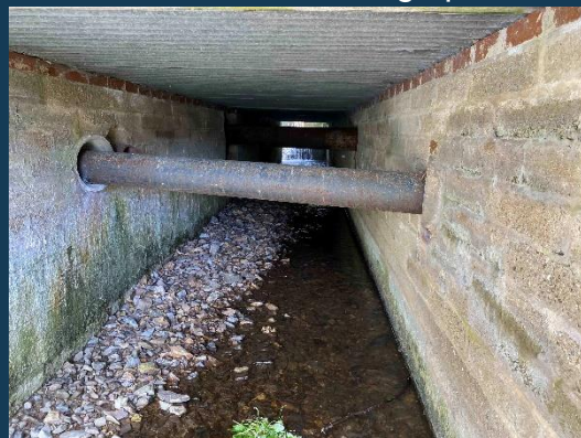
Downstream face, looking upstream:
