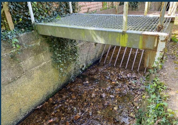
Upstream face, looking downstream:
