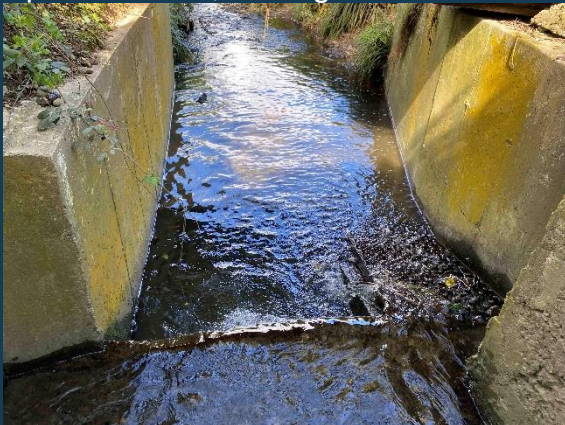
Upstream face, looking downstream:
