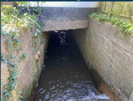
Upstream face, looking downstream:
