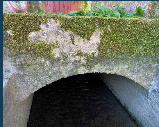
Downstream face, looking upstream:
