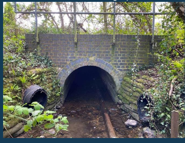
Downstream face, looking upstream:
