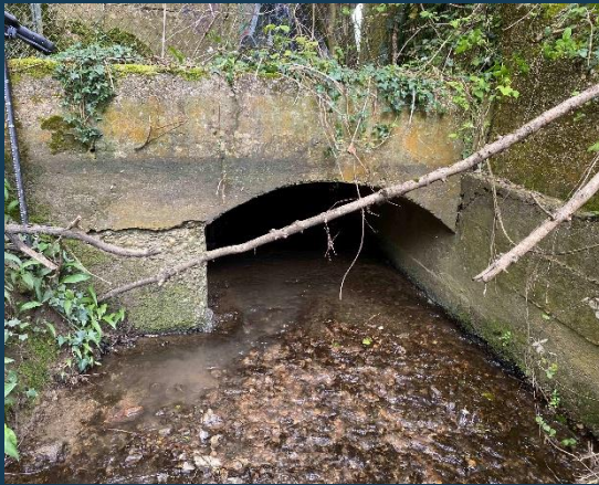
Upstream face, looking downstream:
