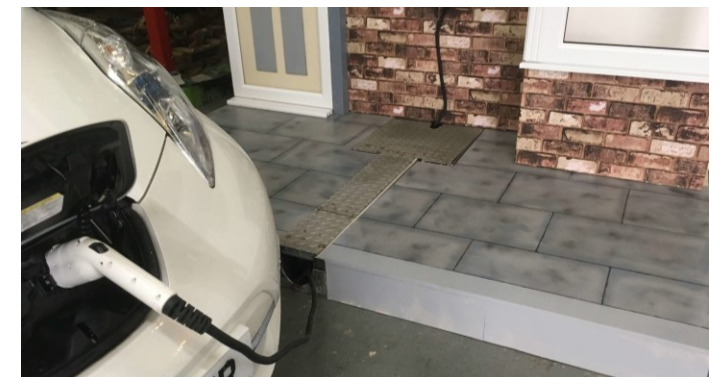
Figure 18 Example of a gully & cable protector
