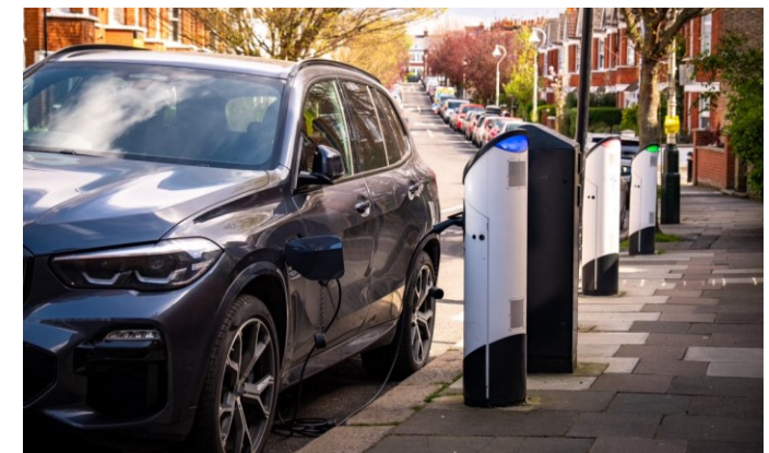
Figure 14 Electric vehicle charge point
