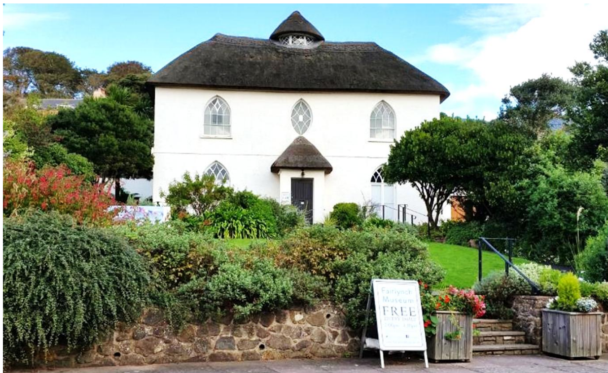
Fairlynch Museum, Budleigh Salterton, example of a 'Cottage Orné building
