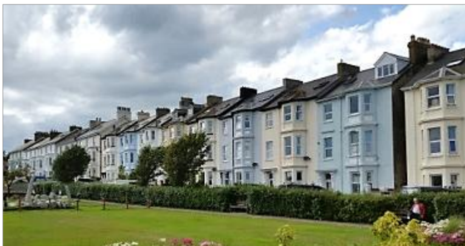
Seaton: 19 th Century 3 storey stucco villas in blocks of 4
