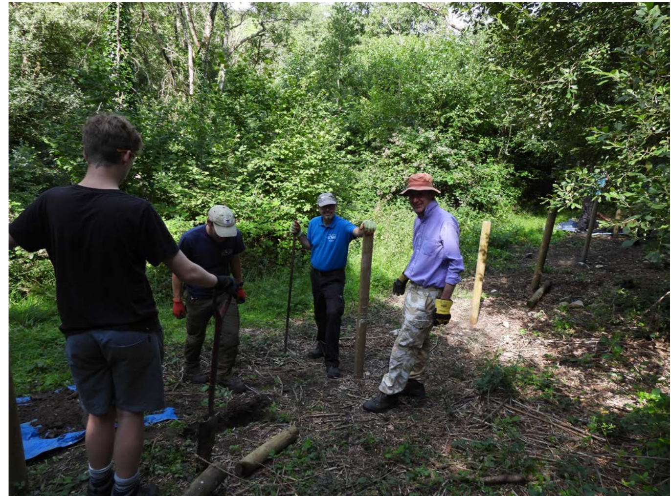
Figure 15. Fence repair at Knapp Copse
