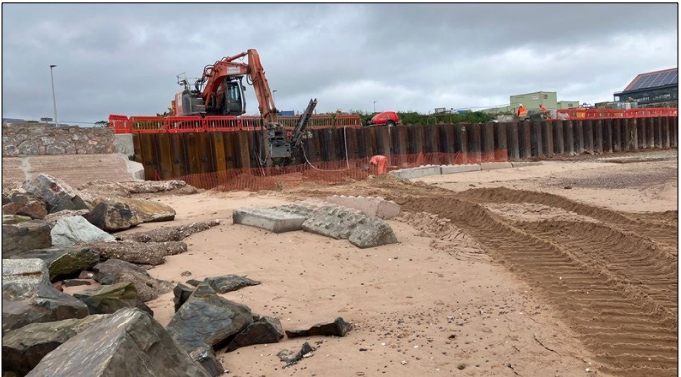
Figure 5: Emergency repairs at Exmouth during Spring 2024.
