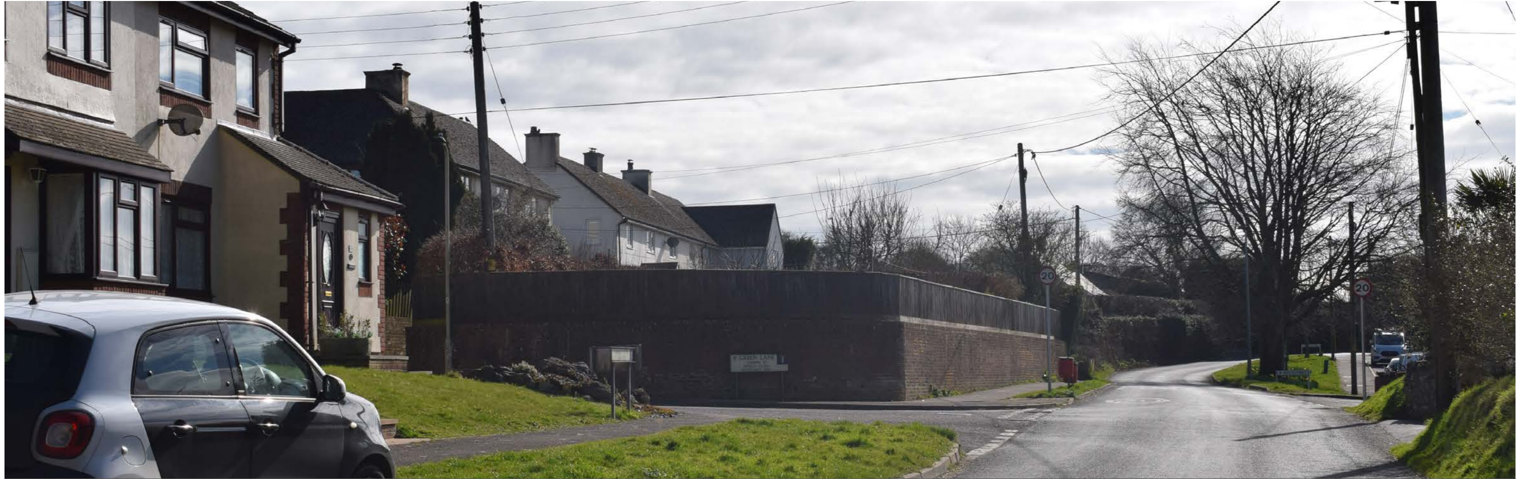
RVP 02 View east towards site from 'The Half Moon Road'
