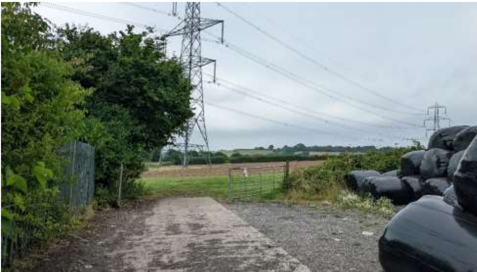
Site existing condition – GH/ED/39b photo taken from the access gate at Northcote Hill
