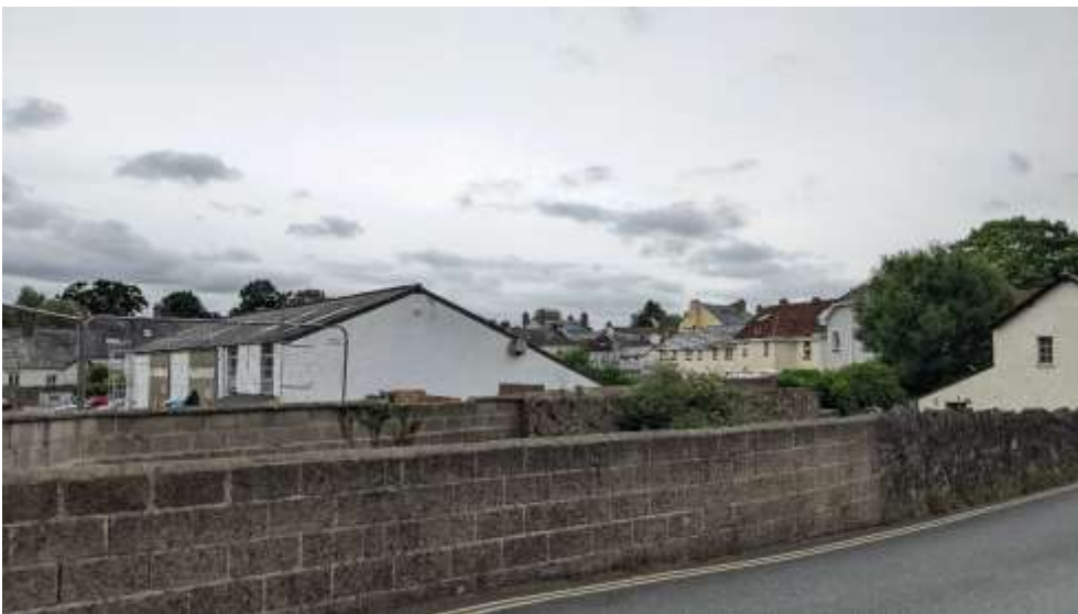
Site existing condition, view from King Street
