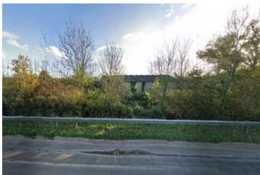
Existing buildings looking south from the A30
