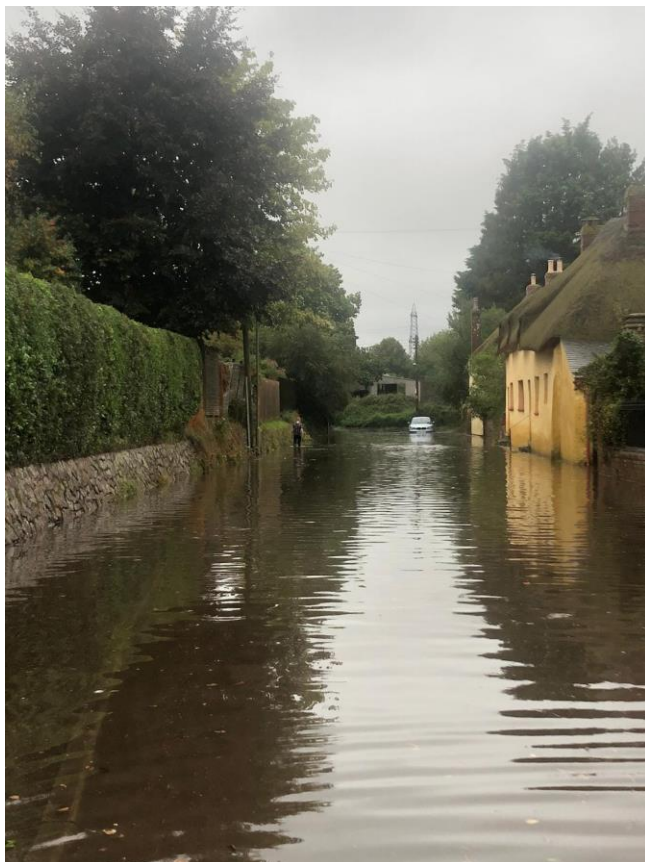
Figure 6: Town End Road under water (17 th September 2023)
