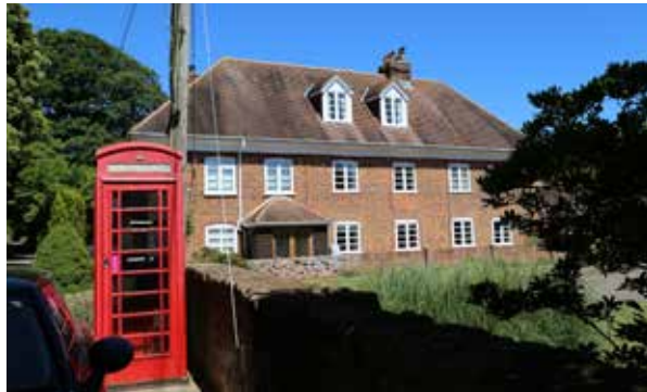
Figure 18: Hipped roof house with clay tiles and overall red brickwork, though with colour variation including darker bricks.
