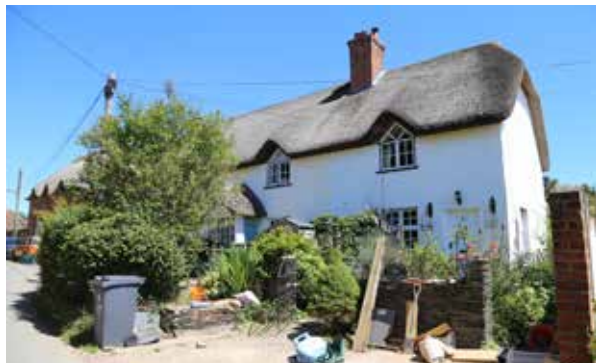
Figure 19: Plastered cob and thatched roof house with eyebrow dormers. Prepared for: Clyst St Mary & Sowton Neighbourhood Plan
