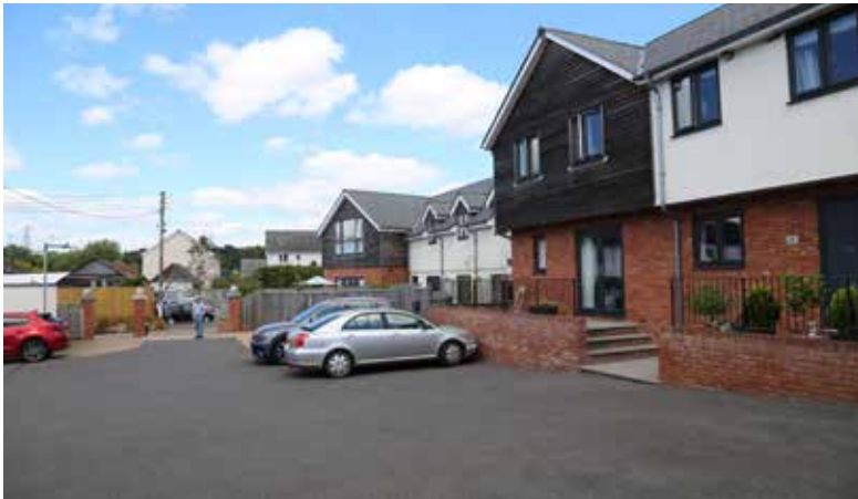
Figure 29: Care needs to be taken when designing car parking within developments. Hard landscaping needs to be minimised in favour of permeable surfaces, soft landscaping can improve the biodiversity as well as outlook for residents and parking should always be to the rear of developments to improve the streetscene.
