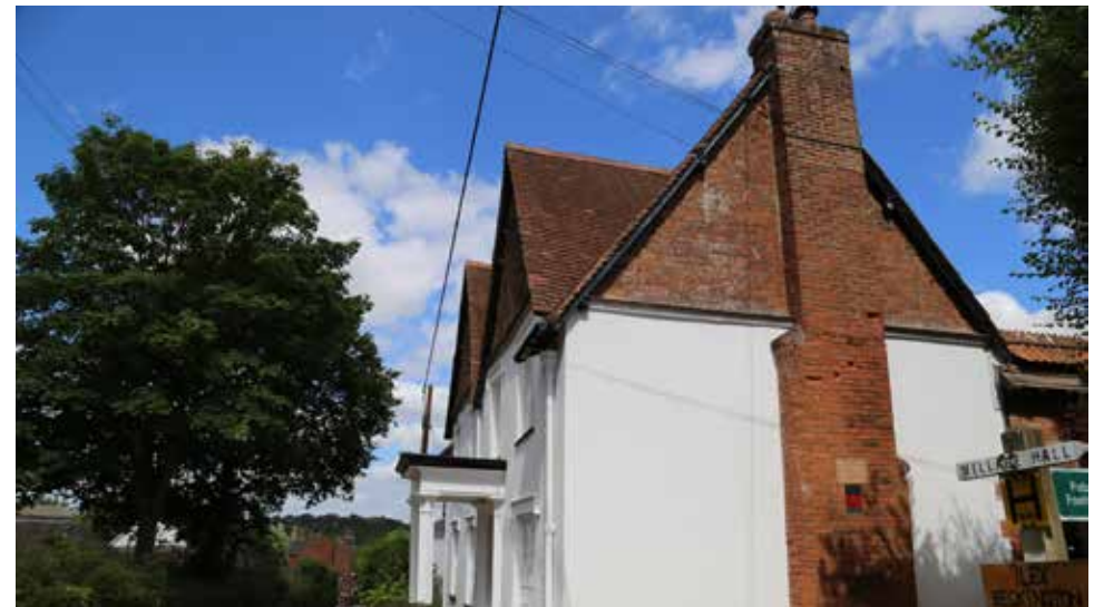
Figure 38: Sensitive new development (top photo) in terms of traditional architecture and village green. Local vernacular materials - red brick, render, slate; windows and dormers in proportion. Add on chimneys should be avoided in favour of full length red brick chimneys on the gable end wall (bottom photo).
