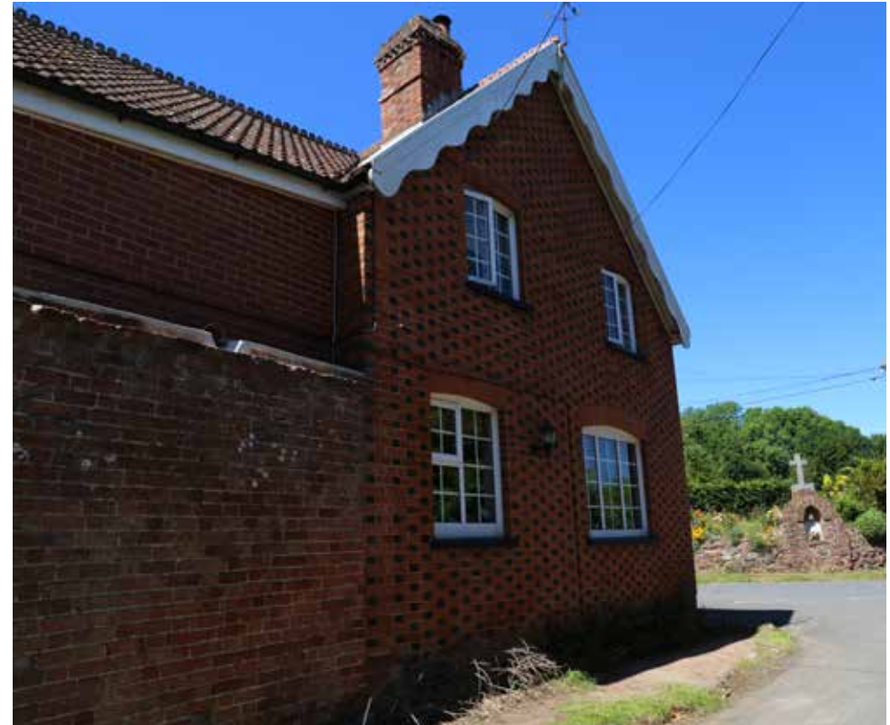
Figure 50: Local example of rear extension in Sowton village, which perhaps could have used reclaimed red brick to blend better with the original building and historic wall.
