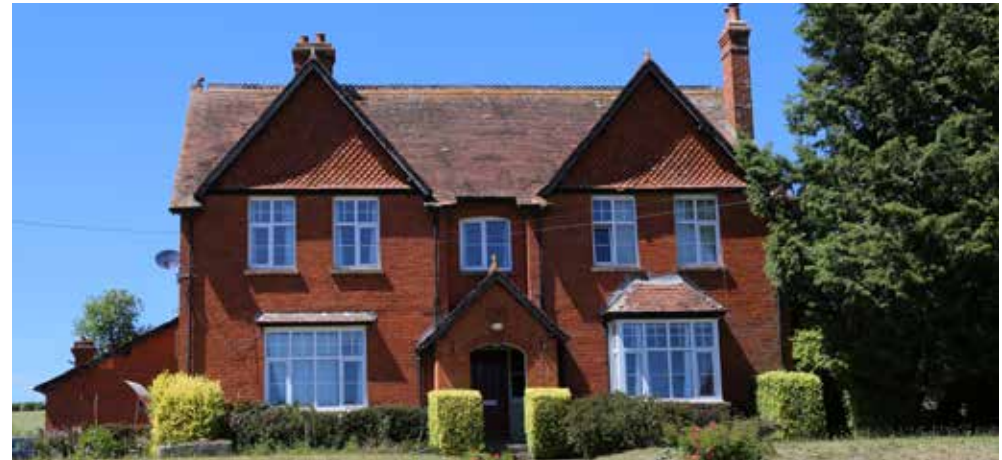
Figure 45: Tile pattern and roof detailing, Sowton.
