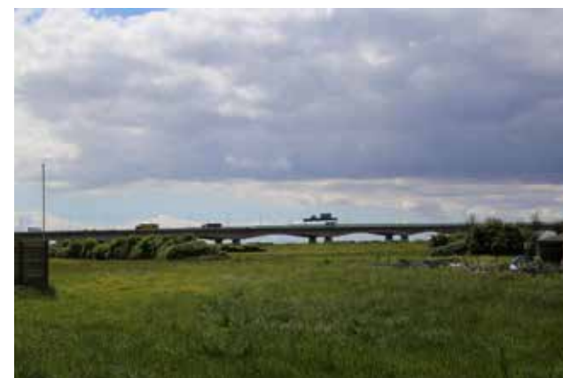
Figure 03: View over floodplain towards elevated section of the M5.
