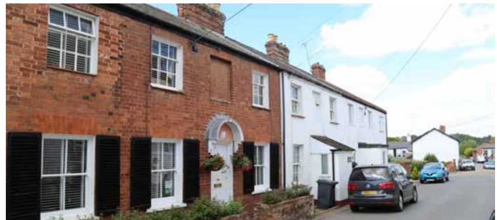
Figure 30: Better example of replacement windows - white hardwood (slimline double glazed preferable) or powder coated aluminium with similar profile to historic windows. NB please consult your local authority for any changes to a listed building.
