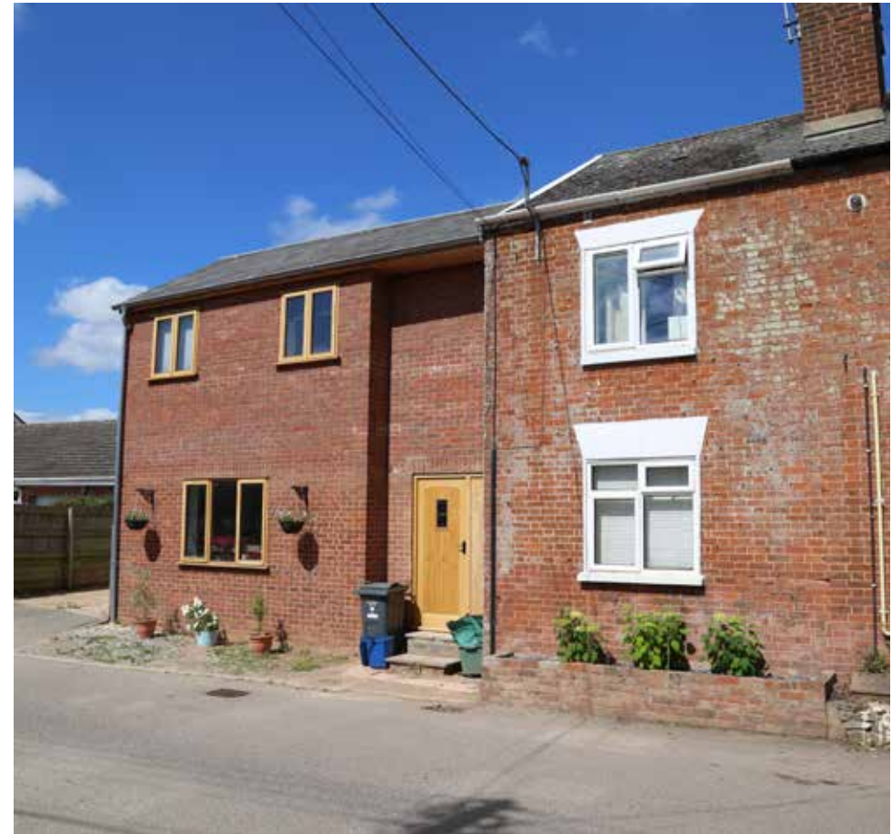
Figure 49: New development onto an existing terrace - important to match window and door dimensions of neighbouring development as well as materials. It is good that the new development in this instance used wooden windows however it would have been better if they were painted white. The window proportions and where they are placed on the front elevation are also not quite correct. It is also peculiar why the new terrace has been set down from the eaves of the neighbouring terrace and not in line forming a continuous and uninterrupted terrace.
