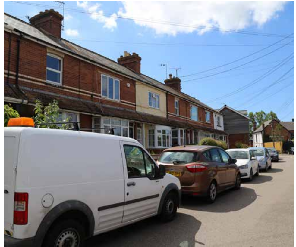
Figure 46: The use of uPVC and the different styles of windows has eroded the historic features on this row of terraces. Going forward traditional wooden sash windows should be encouraged and uPVC with out of proportion profiles and imitation leaded lights avoided.
