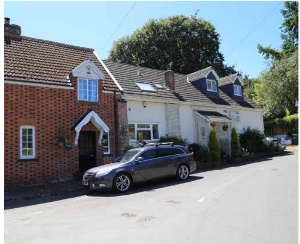
Figure 48: Care should be taken to ensure that materials and the window compositions do not detract from the historic building or Conservation Area. uPVC should be avoided on windows, guttering and barge boards in favour of more traditional materials such as white painted wood for windows/barge boards and black painted metal for rainwater goods. Use casement or sash windows and avoid modern window proportions. New dormer windows should match the existing context so in this example, brick facing, larger casement windows, similar or no barge boards and lead cheeks may have preserved and enhanced the Conservation Area better. Red brick combined with local sandstone, Clyst St Mary.
