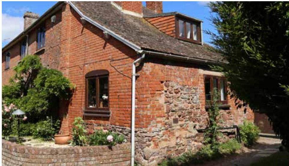
Figure 47: Red brick combined with local sandstone, Clyst St Mary.
