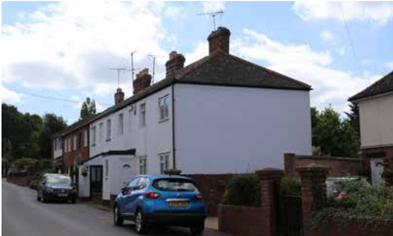
Figure 27: Modern infill and building modifications such as uPVC windows have eroded the streetscene.
