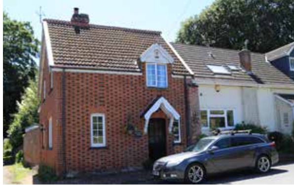
Figure 17: Red and dark brickwork pattern with clay, pantile roof and use of out of character barge board.
