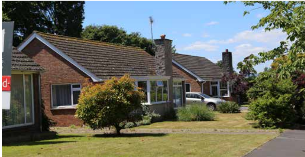
Figure 32: Typical example of mid 20th Century detached bungalow south of A3052 with mix of materials from local vernacular - red brick, stone, slate would be better than concrete tile. Also note generous front gardens and soft landscaping which improves amenity and biodiversity.
