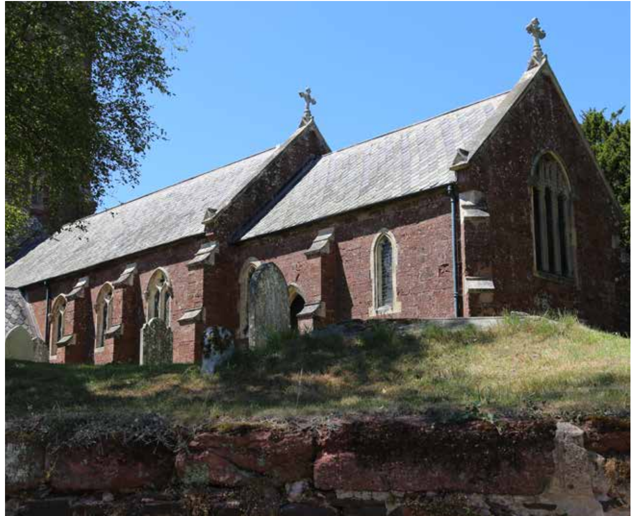
Figure 15: Church of St Michael & All Angels Church, Sowton.
