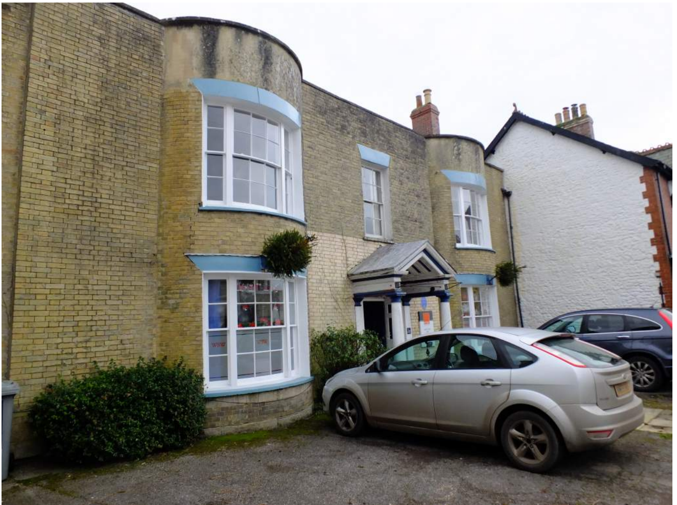
Photo 6: Hey Hop House, Silver Street; part of the Axminster Conservation Area
