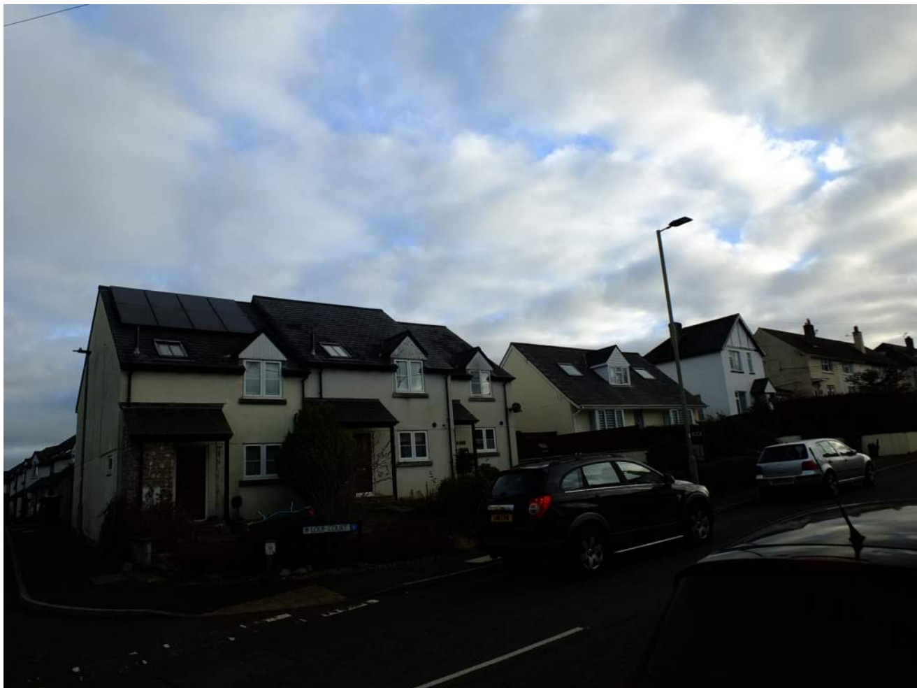
Photo 3: View east from Loup House across Lyme Road toward the Proposed Development.
