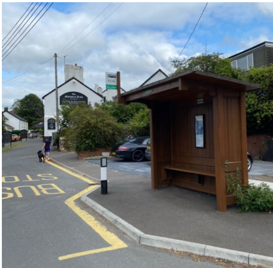
Figure 3-7: Example of a rural bus shelter – joint funded by DCC and Woodbury Parish Council
