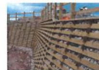
SUPERMARKET: CRIB WALL
