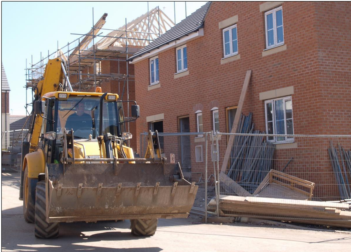
FIGURE 6 Homes under construction.
