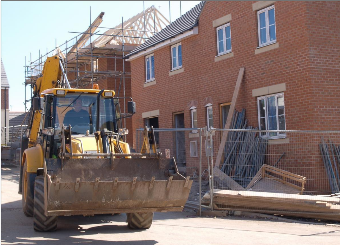
Figure 6. Homes under construction
