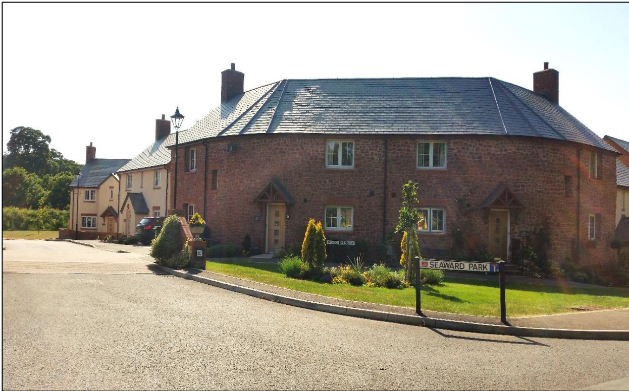
Figure 5. New homes at Clyst St George
