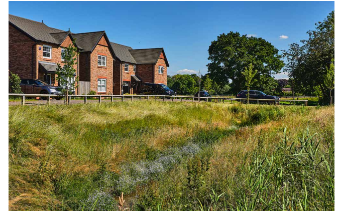
Drainage features are well incorporated into the landscape at Heathfields Farm, Wilmslow (Taylor Wimpey)
