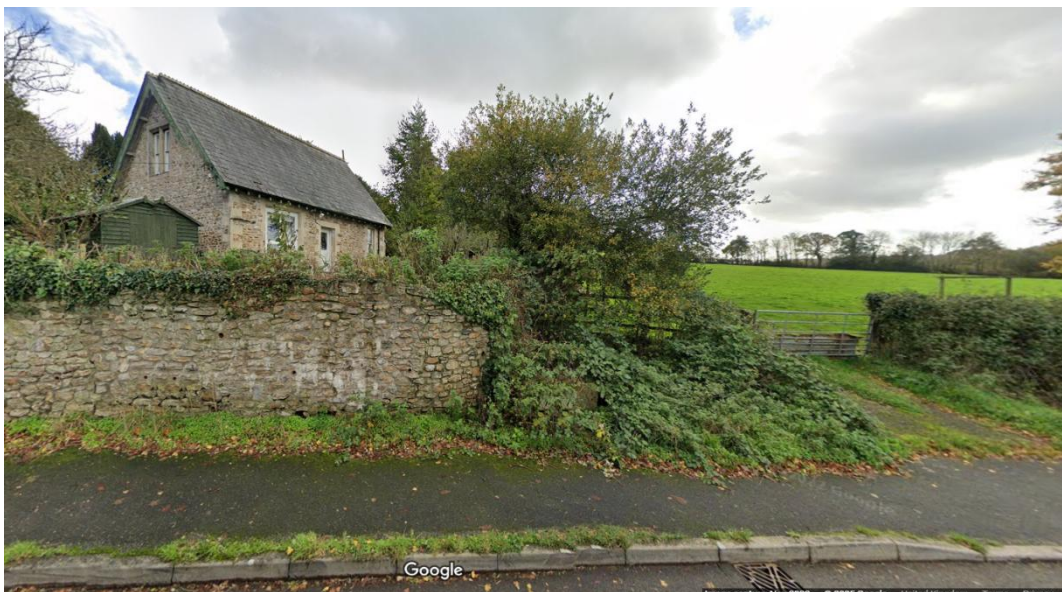
View from Waterleat Ave showing the Former Sexton's House
