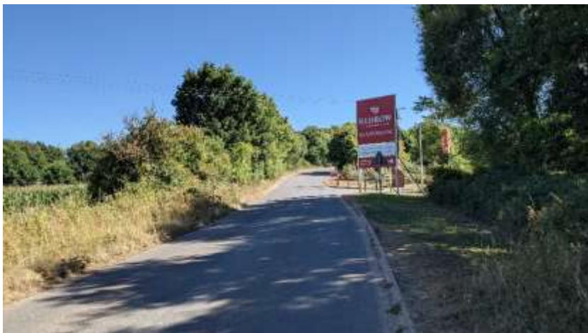
View from Poltimore Road, photo shows the access road.
