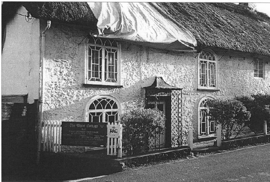
Dolphin Street, White Cottage, good ironwork and woodwork detail to cottage orne, but poorly sited signage and fencing, and decayed thatch
