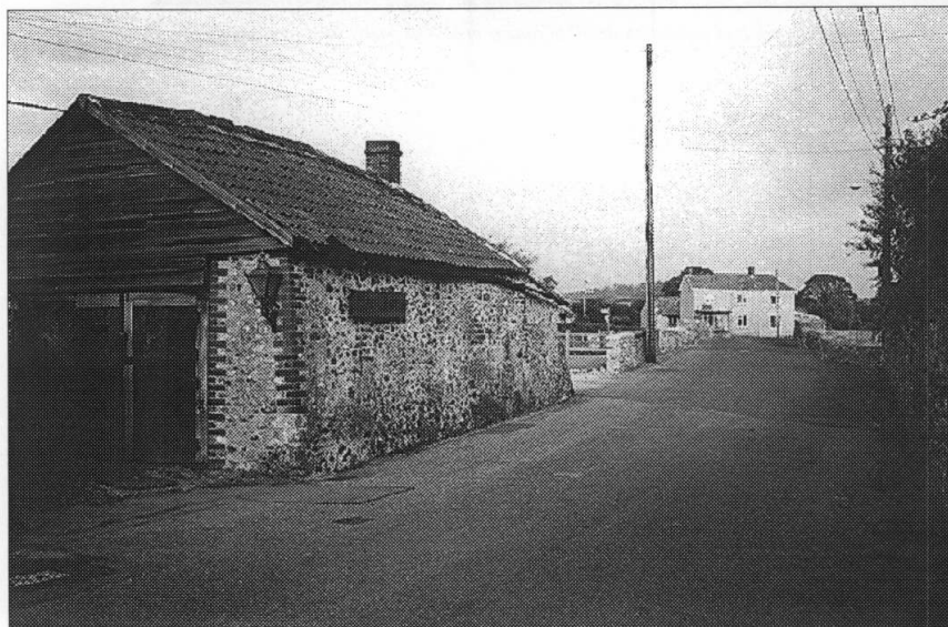
Chantry Bridge, the forge
