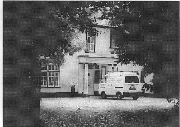
Elysian Fields, Camden has plainer classical detail and some replacement windows
