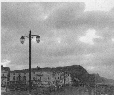
New lamp standards on The Esplanade
