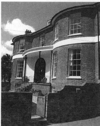
A recently completed restoration of Kennaway House.
