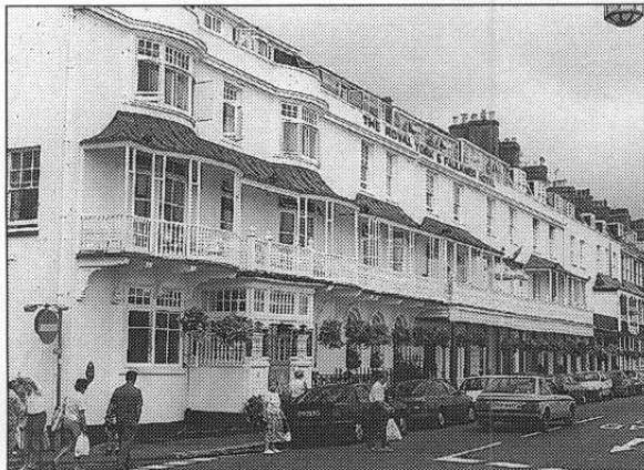
Royal York and Faulkner Hotel with characteristic frontage detail and recently restored porch.
