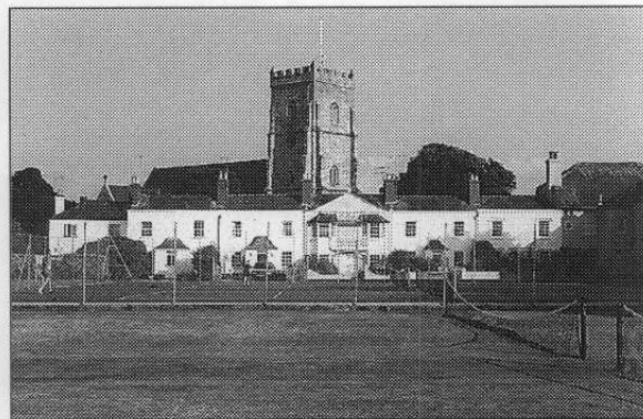
The Parish Church viewed across Coburg Leisure Ground; a dominant landmark and attractive foil to the once symmetrical Amyatt's Terrace.
