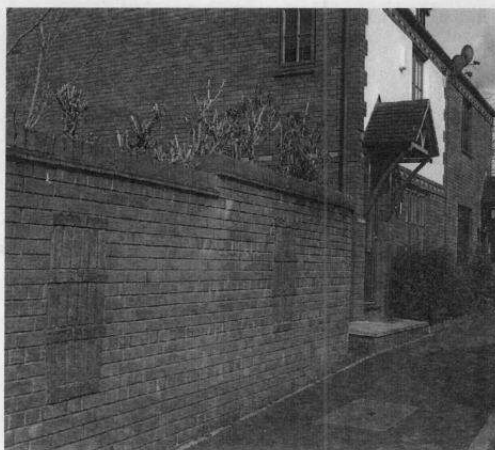
New residential development with strong suburban overtones, yet incorporating a barrel motif in the brick boundary wall.
