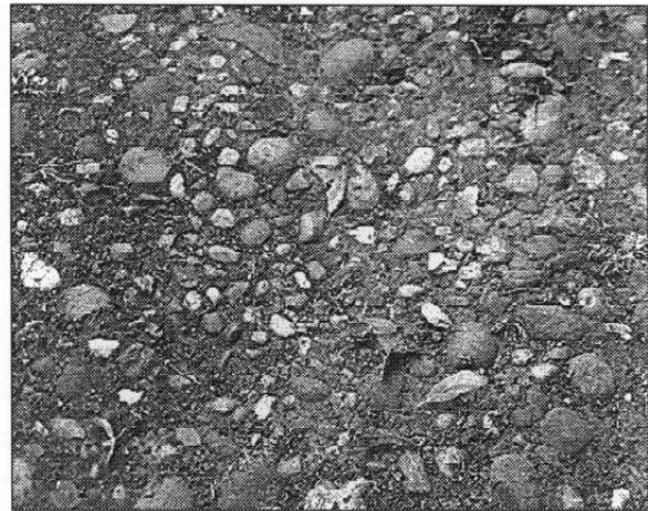
A considerable area of this ground surface exists along the north side of The Square. It has been carefully prepared to give adequate drainage without run-off, and remains firm in wet weather.
