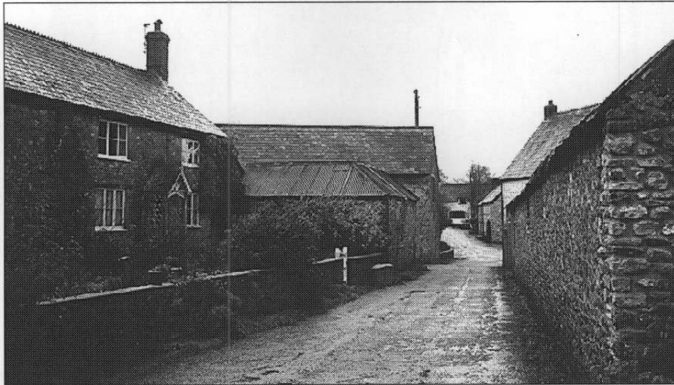
Park Farm outbuildings(right) are to be converted to residential use. Chert stone walls and slate or corrugated iron roofs predominate.
