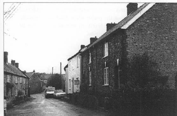
The main village street (Honiton Road) contains 18th and 19th century terraces with chert and slate predominating but with brick dressings and stacks. Casement windows (2,4 or 6 light) are almost universal.
