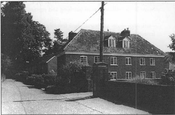
A typical large late 18th century house, now subdivided. The K6 telephone kiosk is prominent. Although overhead power lines are not unduly evident in summer owing to the profusion of foliage, their presence means that trees have to be drastically pruned periodically.
