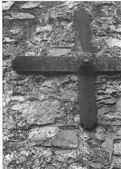
Close-up detail of garden walls in Doatshayne Lane showing typical problems of decayed mortar and frost damaged brickwork (left) and the need to use wall ties to prevent further movement of structurally unsound sections. Here successive applications of cement mortar/render have almost obscured the stonework
