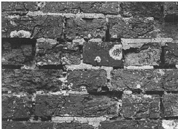
Close-up detail of garden walls in Doatshayne Lane showing typical problems of decayed mortar and frost damaged brickwork (left) and the need to use wall ties to prevent further movement of structurally unsound sections. Here successive applications of cement mortar/render have almost obscured the stonework
