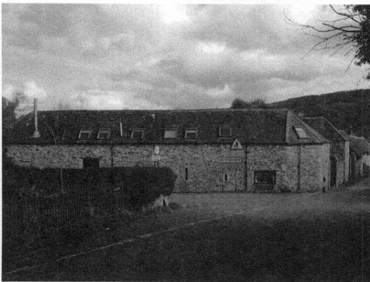
The conversion of barns at Town Farm are prominent within the conservation area with an array of roof lights and flues.
