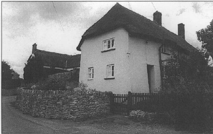
Cob cottage on village outskirts showing tapered walls thickening towards the base. The chert rubble garden wall is typical.
