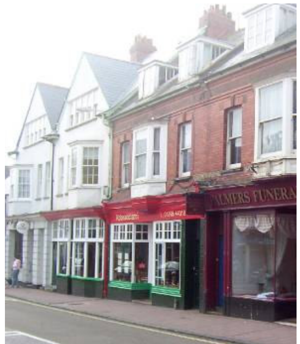
Fore Street shopfronts; there is a good survival of traditional shopfronts with good plain lettering.
