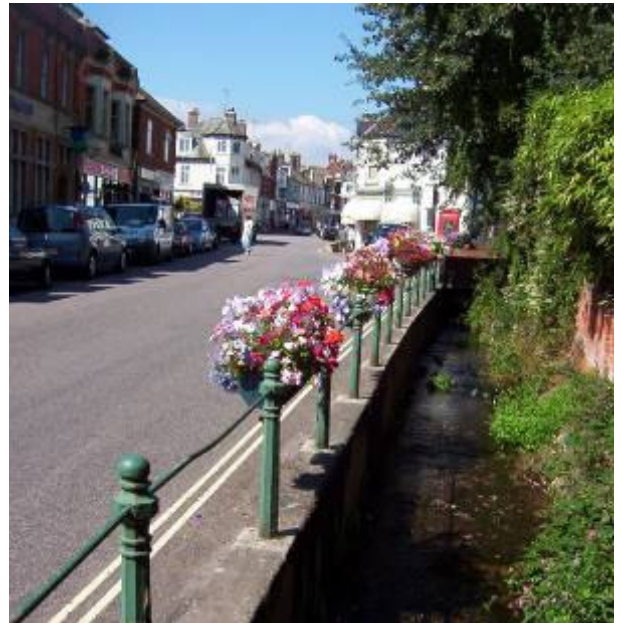
Fore Street: the stream, footbridges and recently introduced railings create a pleasing foil to commercial frontages.
