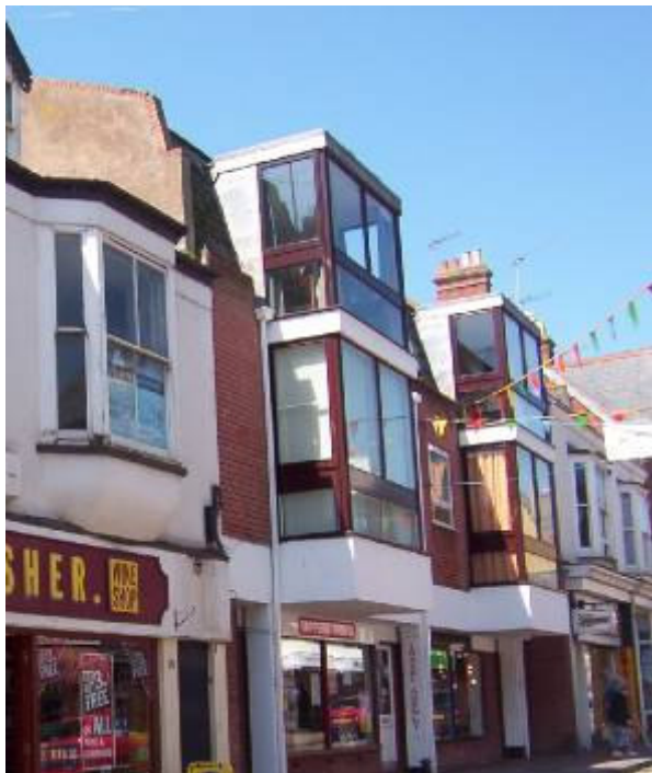
Fore Street; updated frontages or new infill has tended to undermine the historic environment, although in time such development may come to be seen as representing a period style.
