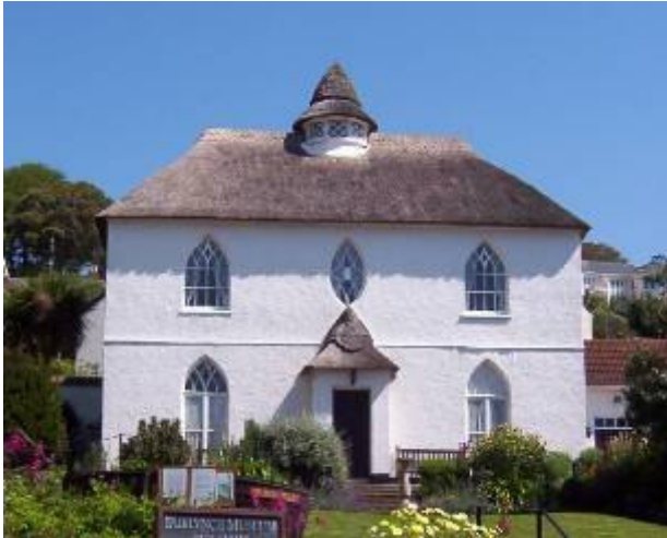
Fairlynch; Gothic window details and thatch, typical of the "cottage orne" tradition.
