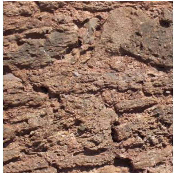
Local sandstone walls enclosing gardens in Cliff Terrace.
