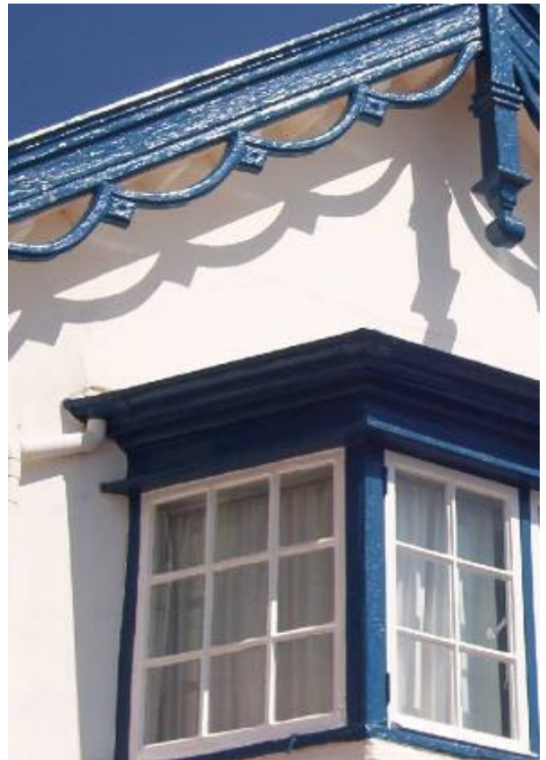
Decorative bargeboards, common on nineteenth century properties.
