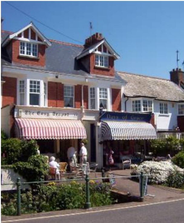
Fore Street (north side); a typical late 19th century group with added shopfronts
