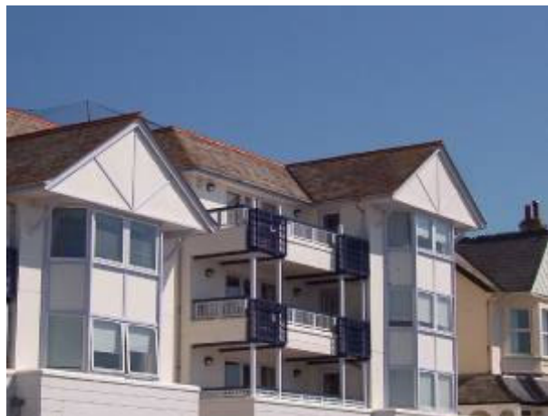
Marine Parade: seafront housing, mainly early to late 20th century. The pale shades of slate (above) are probably Cornish in origin.
