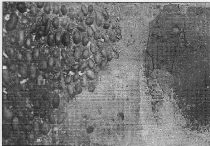
There is an abundance of local building materials in Axminster, not all in a good state of repair. Soft liassic limestone, difficult to repoint (above left), Beerstone dressings beginning to spall (below left) Ham Hill stone dressings and chert rubblestone infill (below right).
