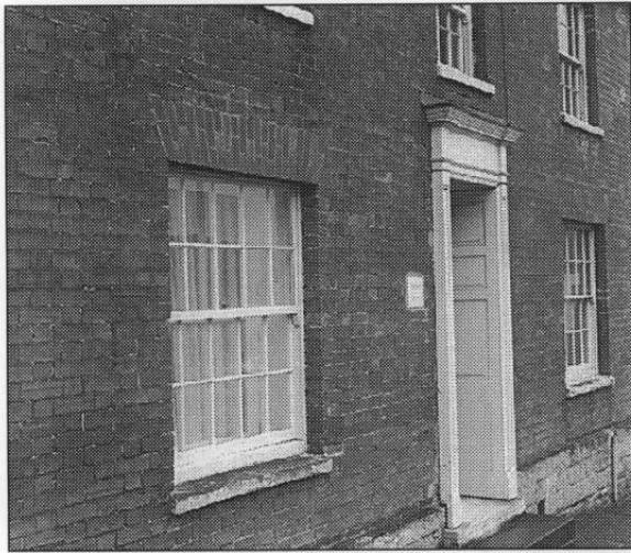
Chard Street; a good example of hand-made brick and replacement when necessary needs particular care. Note stone footings.
