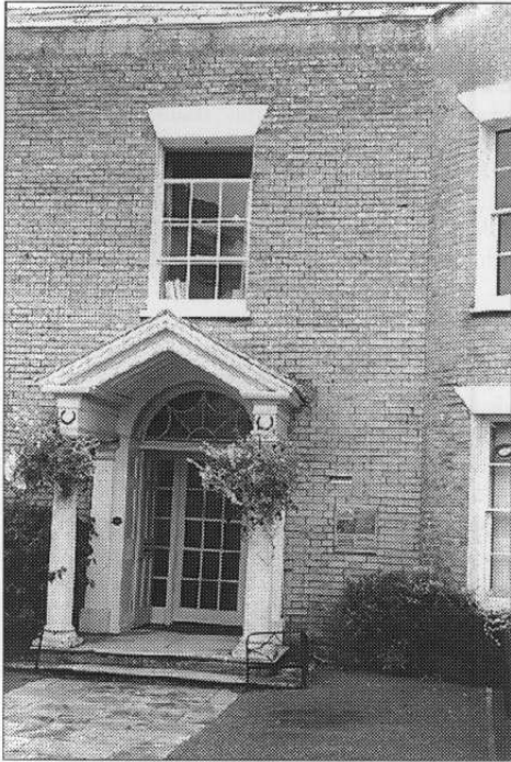
Former town house (now offices) in Silver Street. Mellow stone or brickwork are a particular Axminster feature and this building is faced with cream mathematical tiles.
