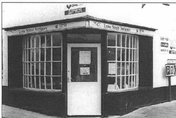
Fine late 18th - early 19th century shopfronts; South Street/Lyme Street (above); Chard Street (right)
