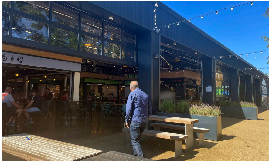
Figures 12 & 13. The Shed, in the new community at Whitehill and Borden, adapts an agricultural portal-frame shed to house small business units. It is a popular meeting place for residents and an important, easily recognisable part of the community's identity.
