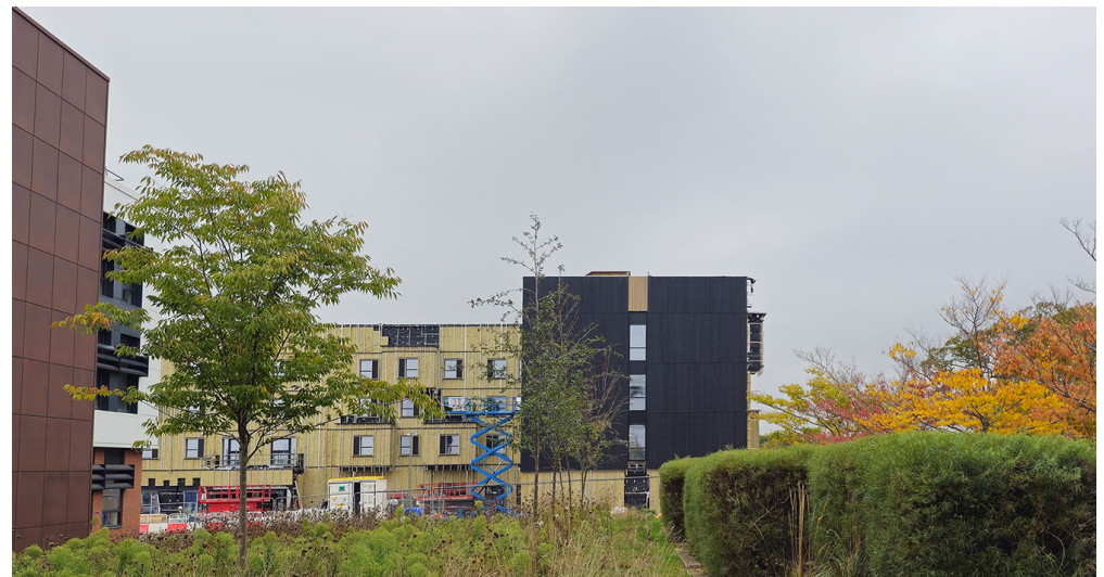
Figure 26. The new hotel currently under construction at the Science Park is highly ambitious in its use of sustainable technology, with a solar facade and solar roof expected to produce more energy than the building uses over the course of a year, and sustainable construction meeting RIBA 2030 embodied energy targets.
