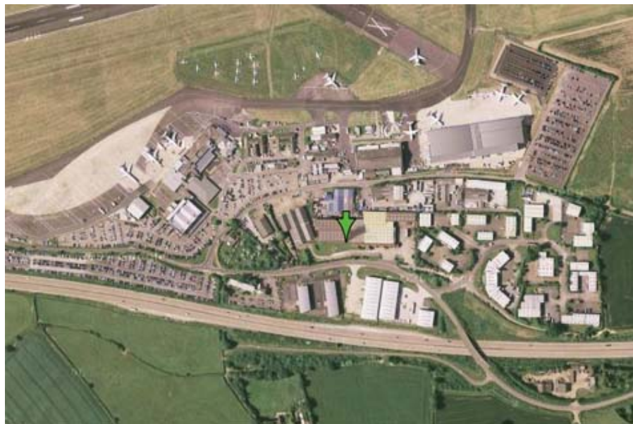
Figure 55, More detailed image of the existing airport terminal. The current proposal is to develop a new terminal building on the west side of the existing plot.
