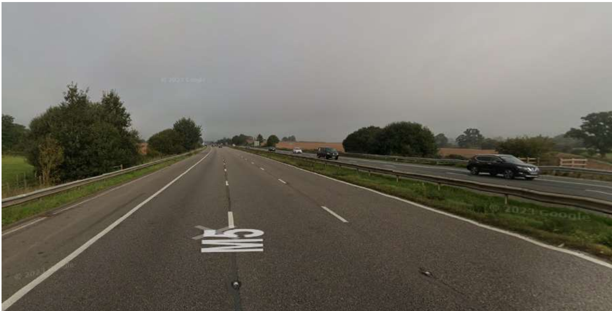
M5 looking north from the south of the site. It can be seen on both sides of the road
