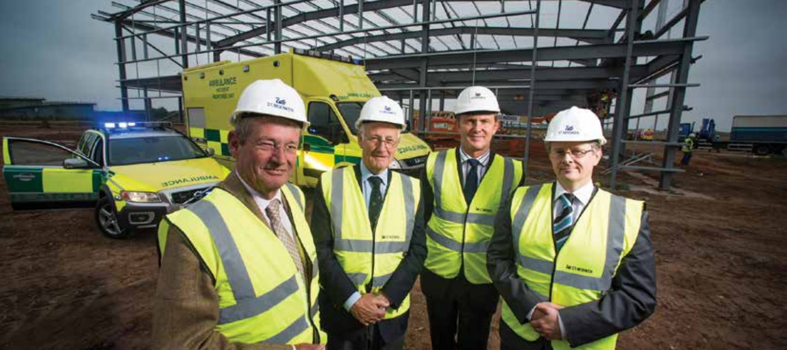
Site of the new ambulance special operations centre at Skypark
