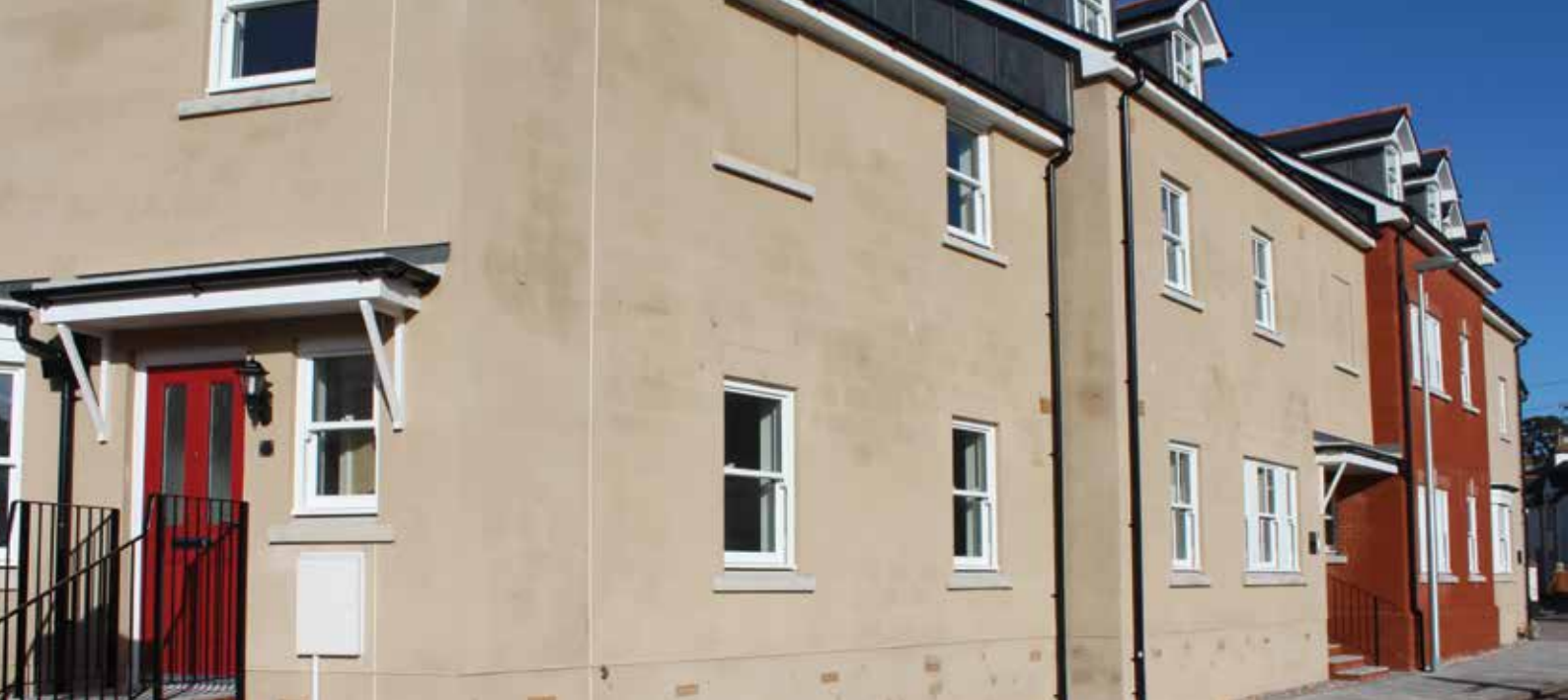
Twelve new affordable flats in Mill Street in Sidmouth
