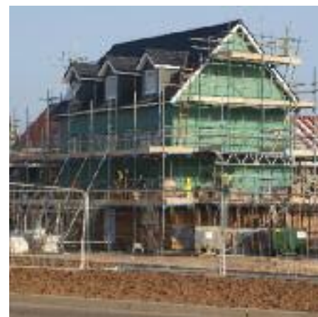
New homes being built at Cranbrook
