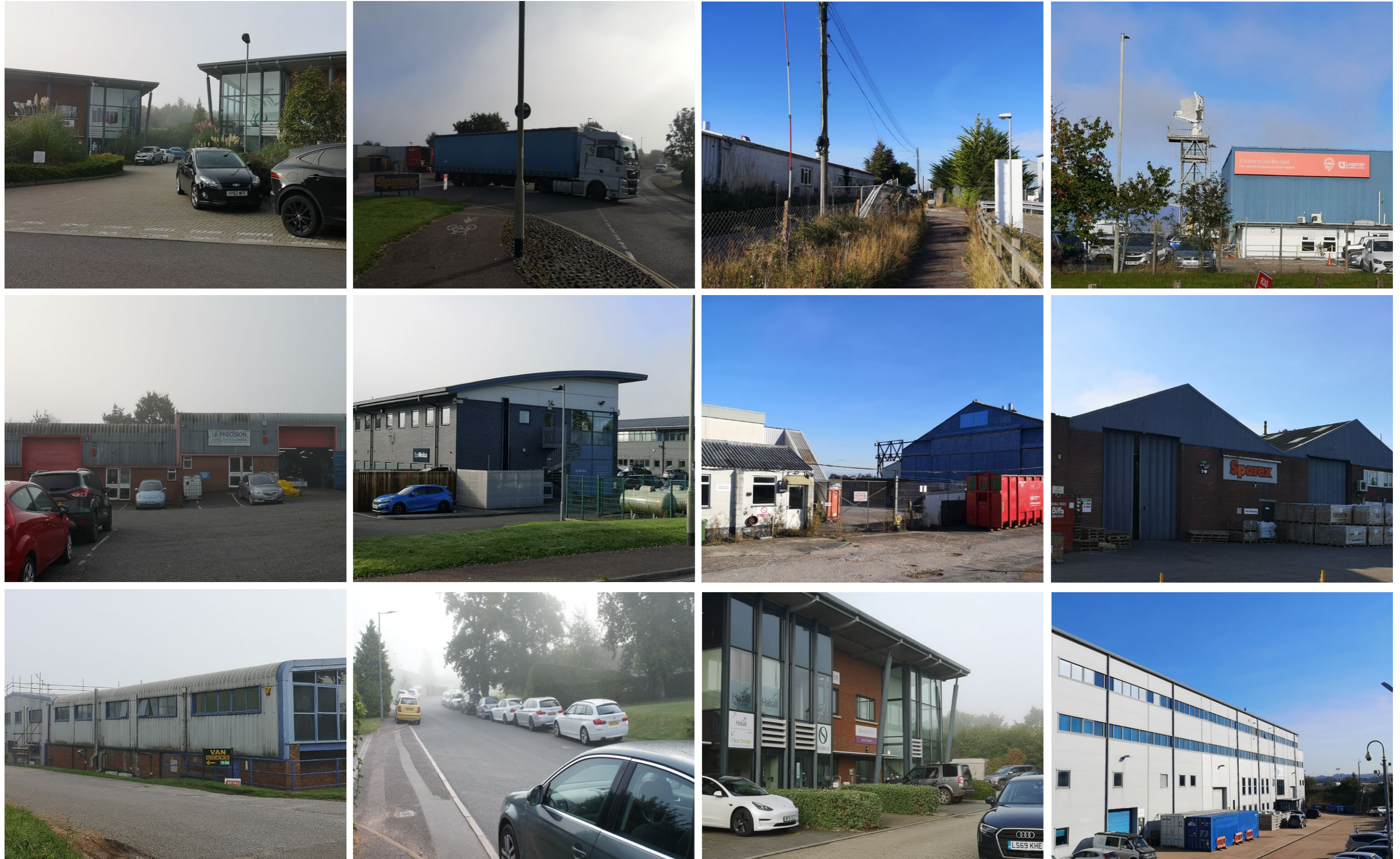
Above: Photographs of existing Exeter Business Park
