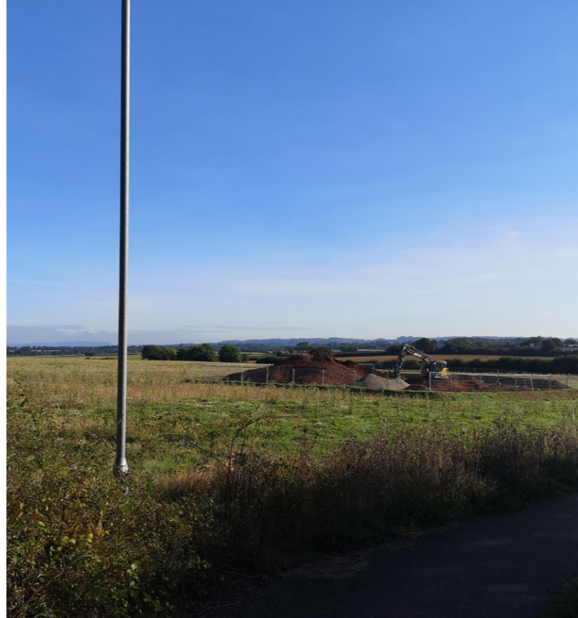
Above: View from Long Lane to Site
