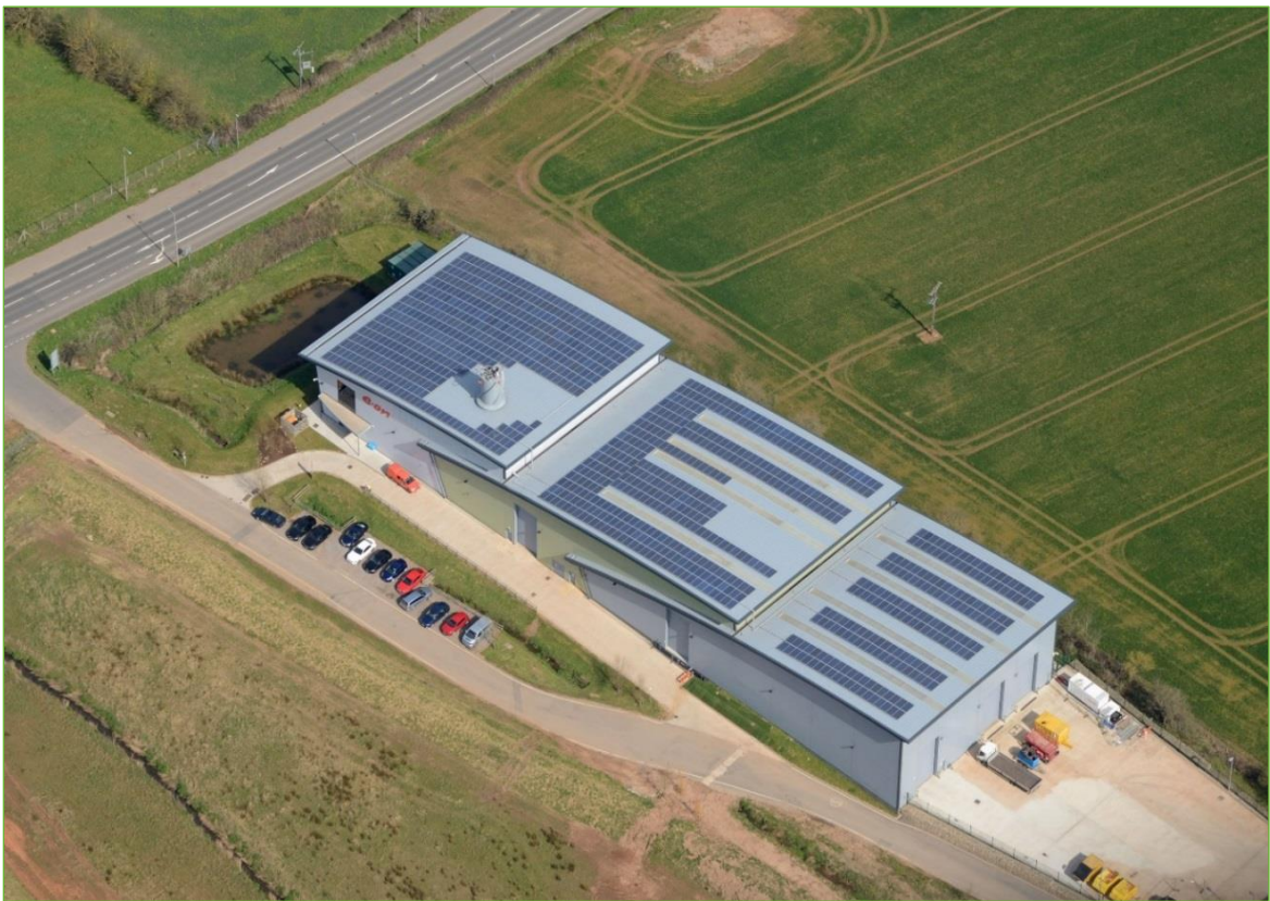
Figure 5 - Aerial photograph of the existing Energy Centre which serves Cranbrook on a district heating network. The land to the right of the energy centre is the western extent of the Treasbare Expansion Area. (Image credit: Still Imaging)
