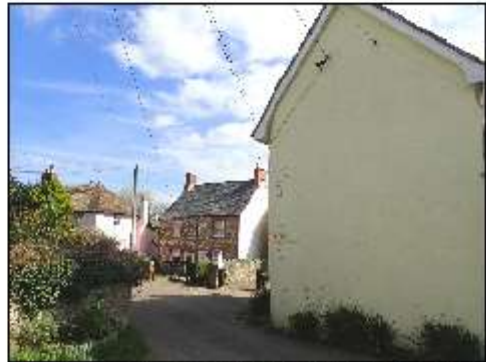
The Hill - an old connecting road to the A35. Lorries struggle to get through the 'dog leg'. Note damage on building
