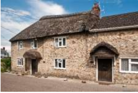
Traditional chert rubblestone laid randomly, sometimes rendered or painted
