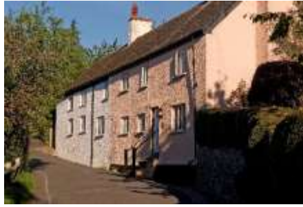
Traditional chert rubblestone laid randomly, sometimes rendered or painted
