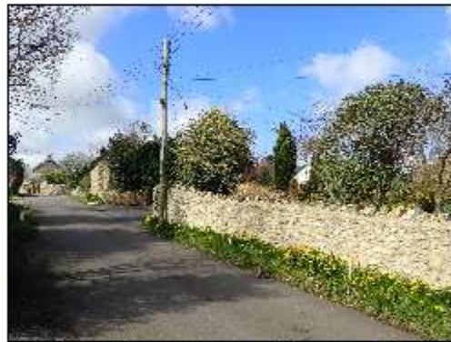
Recently renovated rumble stone wall
