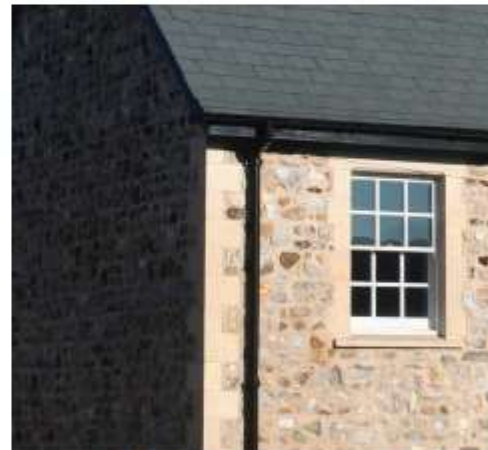
Plain and simple fascia board with dark coloured gutters and downpipes are generally less obtrusive
