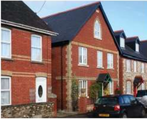
New properties (centre and right) fit into the street scene by having similar proportions to older neighbours (left)
