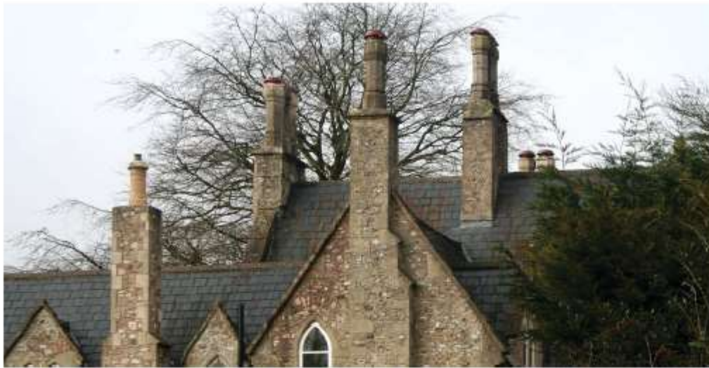
This Victorian house in Bishopswood shows that chimney stacks can be interesting features in their own right
