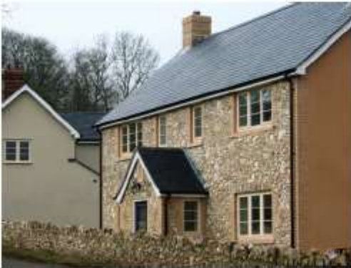
House under construction in the Blackdown Hills
