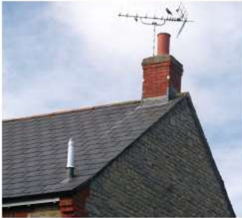
Characteristic gable end roof under modern slate
