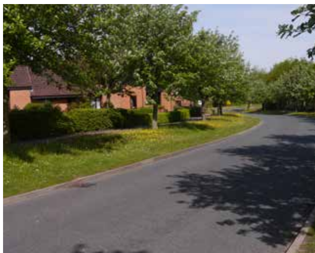
Figure 9 Trees provide partial shade along a flower rich verge. This verge could have been configured to take run-off water from the road.
