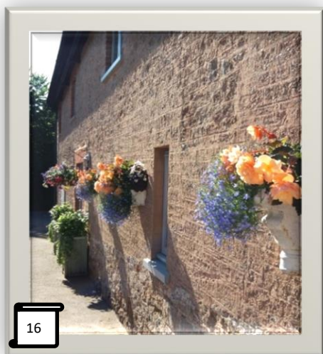
Mid-C19 barn conversion, Ottery Street
