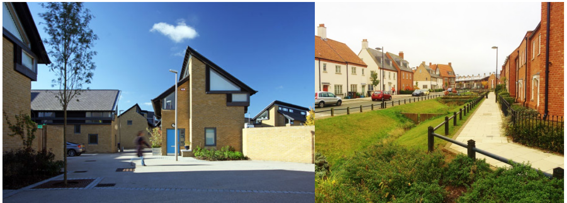
New Hall, Harlow, Essex
