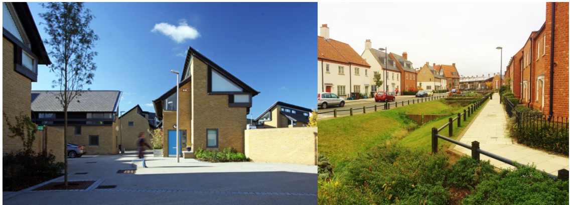
New Hall, Harlow, Essex
