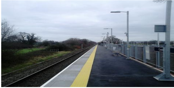
Cranbrook Station, Devon (N.B Single Track)
