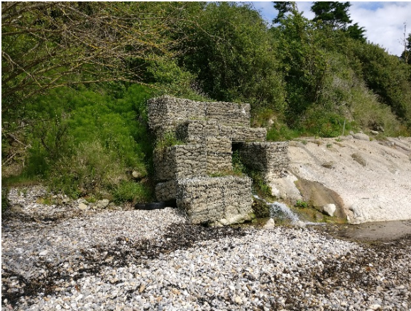
Gabion baskets protecting an outfall
