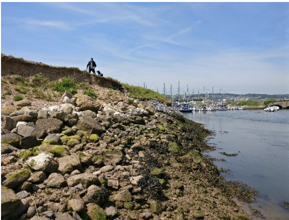
Larger cobbles protecting the back of the spit where cliffing and erosion has occurred
