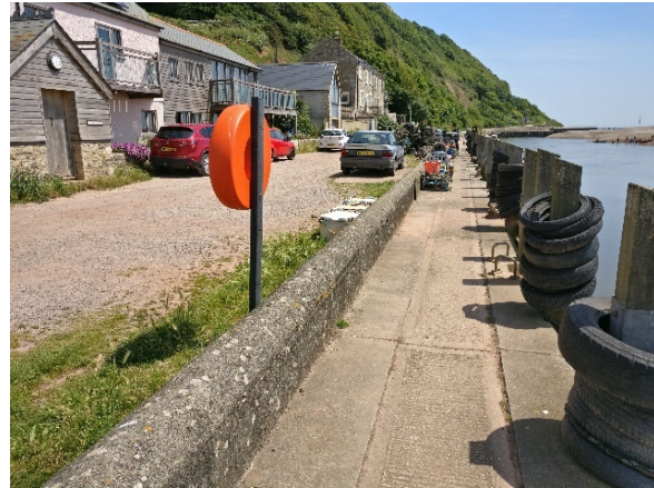
Concrete slab and short flood wall
