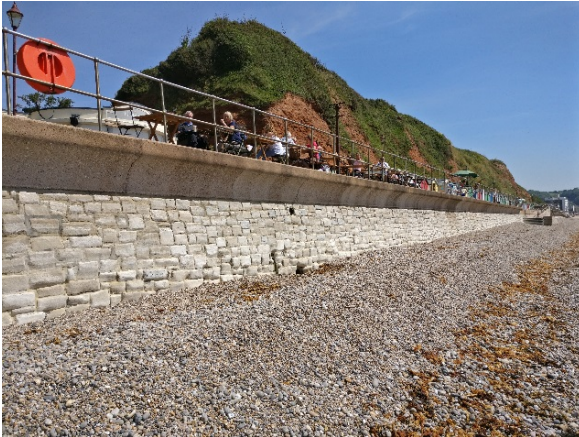
Stone block seawall topped with concrete recurve
