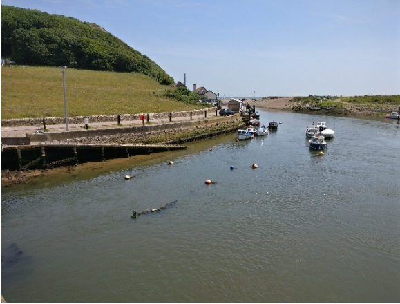
Composite flood defence with timber slipway
