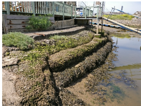
Gabion structures forming steeper defence profile
