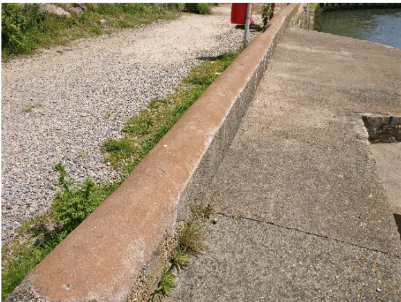
Patch repairs to the concrete flood wall
