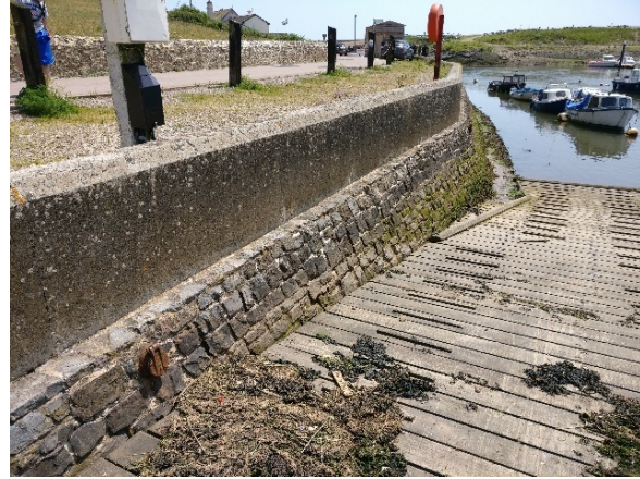
Composite structure with stone block lower wall and concrete upper wall
