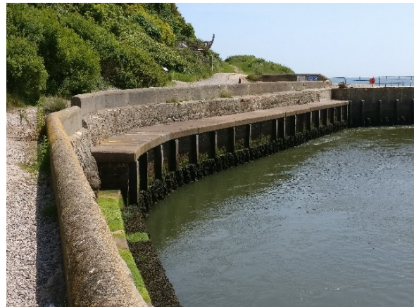
Concrete platform connected to the seawall close to the river mouth
