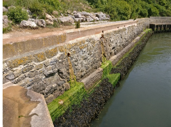
Patch repairs to the upper section of stone block wall
