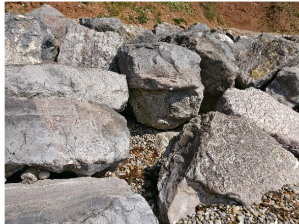
Large voids present within the structure
