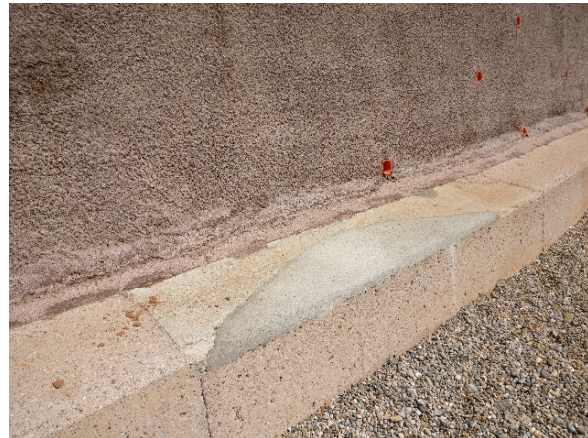
Patch repairs to concrete toe
