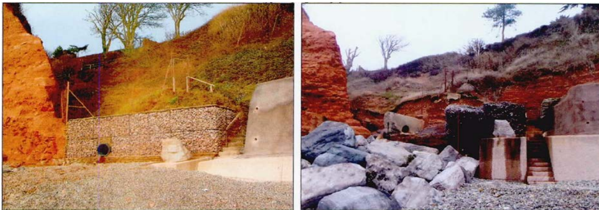
Figure 2-8 Construction photograph (2005) alongside the inspection photograph (2015) Source: David Roche GeoConsulting (2015)
