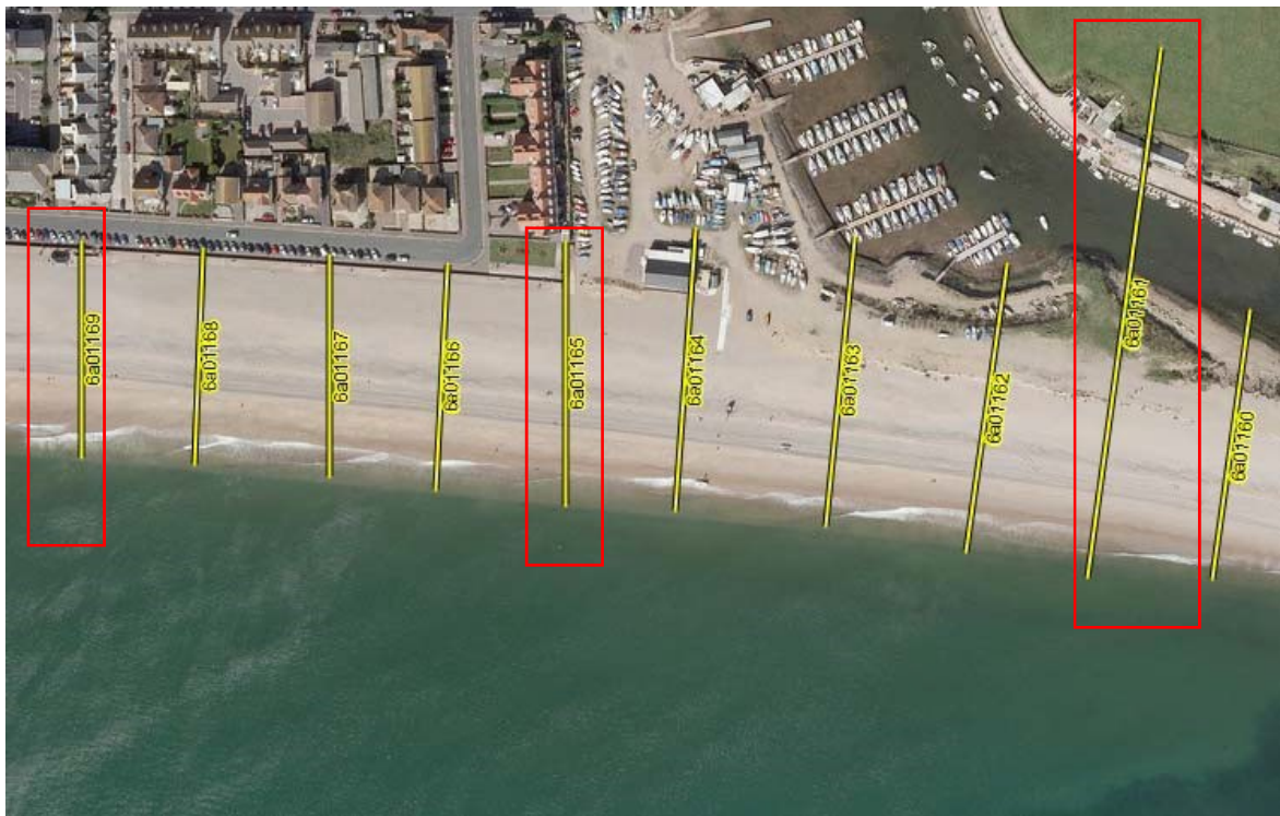
Figure 4.17 Map showing locations of eroding profiles at eastern the end of Seaton, including 6a01169, 6a01165 and 6a01161 Source: Photo Channel Coast Observatory, 2009
