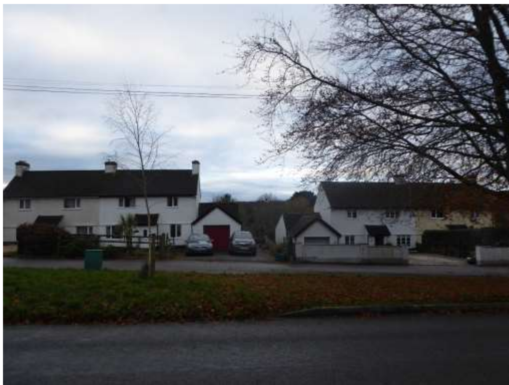
View from access across main road (looking opposite image above)
