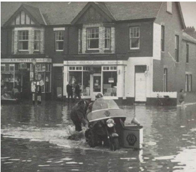
Junction of Hartopp Road and Exeter Road 1960
