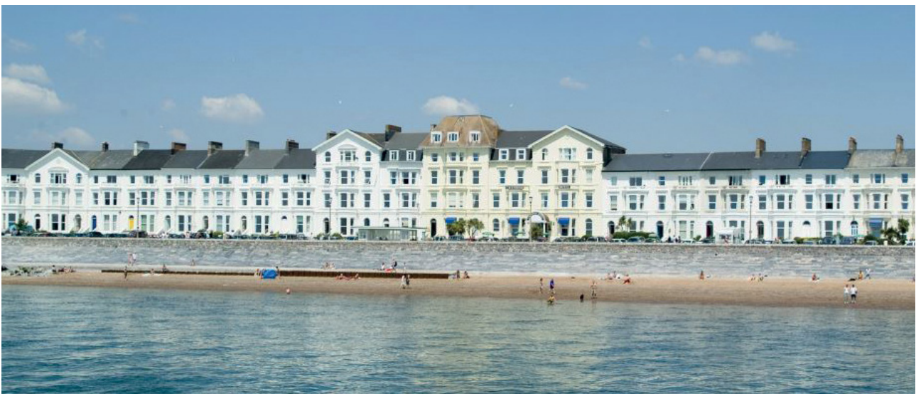
Smeaton's sea wall finished 1842
