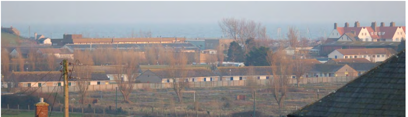
Looking South East across the Seaton Regeneration Area towards the sea.
