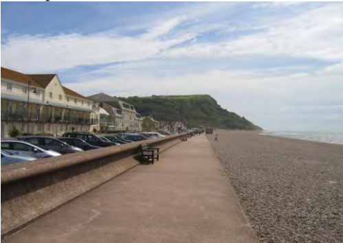
Seawall and Promenade.
