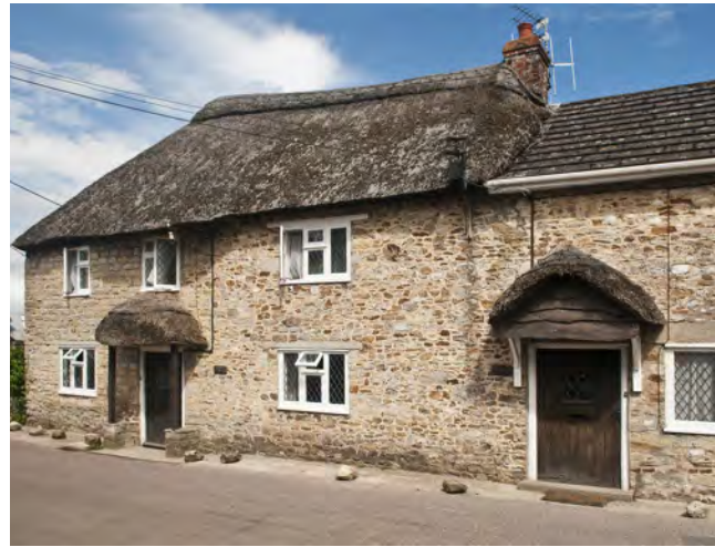
Ashes Farm (above) - rubblestone under thatch, and The Old Bakery and Gowrie House - coated rubblestone
