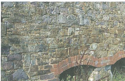
BEER DAIRY BARN This wall shows two quite different builds, in two different kinds of stone. The lower build, just above the brick arches, is remarkably fine. The build above is of mixed stone (including 'Thorverton Blue') and is less regular in construction.
