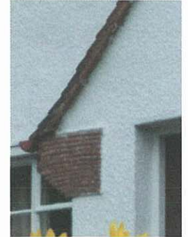
BROADPARK Tiled corbels enliven walls under eaves and on porches in this house and others nearby.
