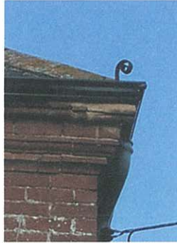
CHAMBERLAINS Fine Victorian brick corbelling
