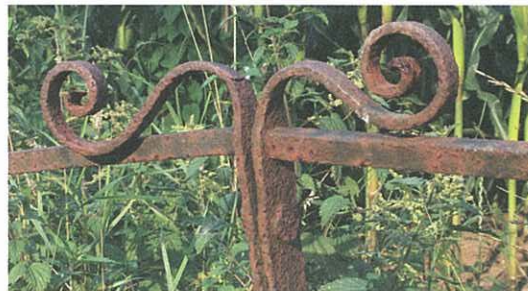
MAIN STREET The decorative wrought-iron fence, now sadly decayed, along the western side of 'The Green', is hand-forged without welding: scroll-tips are delicately flattened rather than chopped off. The fence, not tall or strong enough to restrain cattle, may have marked the social importance of a once-public space.
