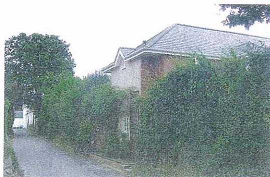
A building integrated with its surroundings
