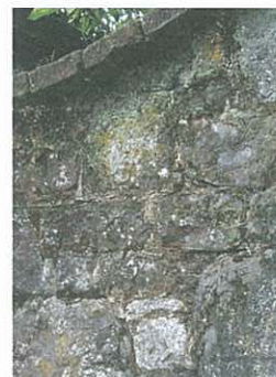
MAIN STREET Volcanic trap in a wall by Bootham House. The stones are tightly packed in random form, the mortar recessed.
